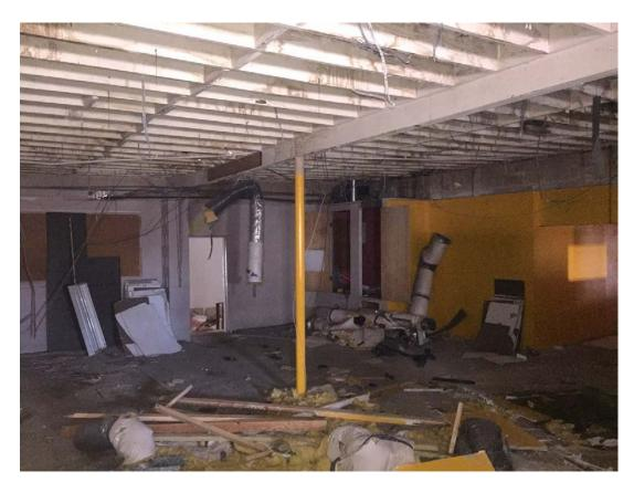
Above is another picture of the interior of the building. Again, portions of the ceiling have fallen onto the first floor. There is ductwork, debris and hazardous materials throughout the building. There is also evidence that animals of some sort have gotten into the building.
