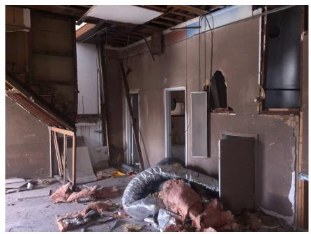
The interior of the building is in total disrepair. In the picture above, part of the ceiling has fallen onto the first floor and there is ductwork that has fallen as well. There is no heat or air in the building. The staircase to the second story is pictured on the left. The bottom portion of the stairs are no longer present providing no access to the second story.
